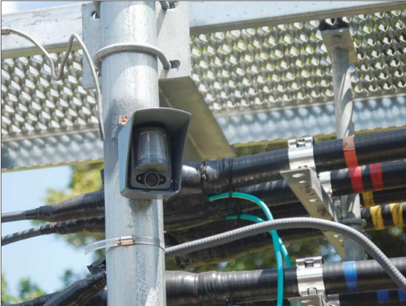
**This camera gives a straight view from the cable tray looking outward, revealing any possible intruders to viewers at the security monitoring center. Metal thieves might be attracted by the copper in the wires shown here covered with green insulation.**
